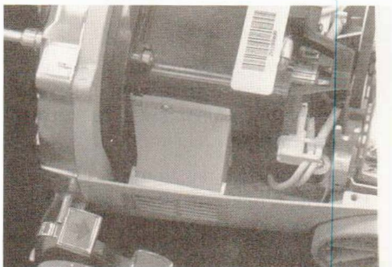
Figure 13. Exhaust Duct and Grill Removal
